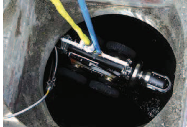
Figure 5.7: Lowering the crawler into a manhole
